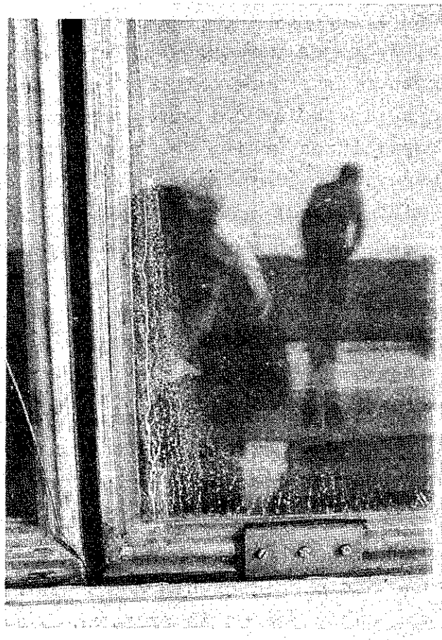
Fig. 2 Outgassing from insulation or from sealant.
